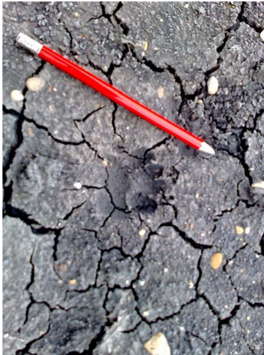
Photograph 2: Footprints close landfill area.
